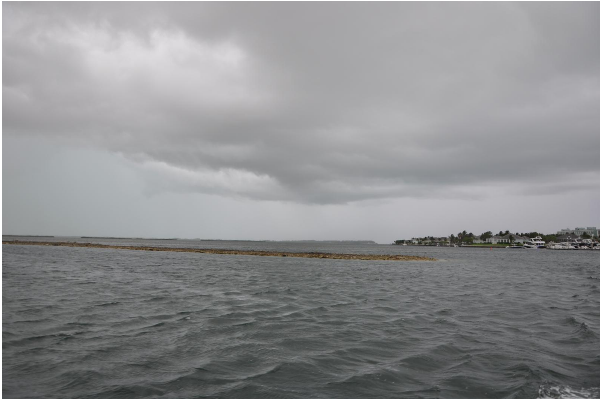
Fig.2: Photo of exposed embankment
