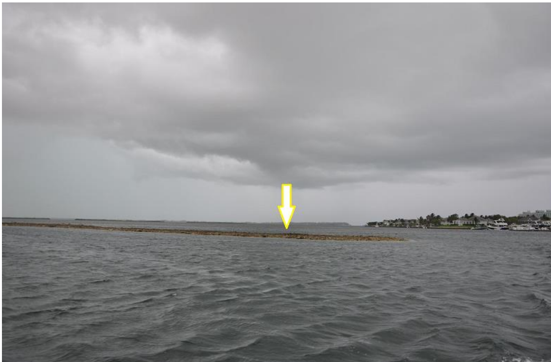
Fig.1: Photo of exposed embankment
