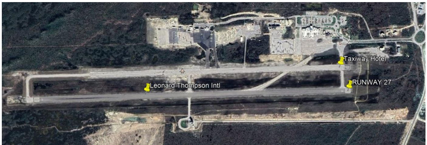
(Google Earth image of Leonard Thompson International Airport, Marsh Harbour, Abaco)
